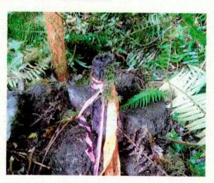
Referenced out the Iron Pipe and set a 30" Iron Pipe with 3" dia. Brass Cap marked as shown above in its position. Set a 12" dia. plastic ring with 120 lbs. of concrete around monument. Replaced the mound of stone and layed the found pipe, found stone and found white painted cedar post on the North side of the monument. Set a 72" Hat Section Post 3.0' North of the monument.
