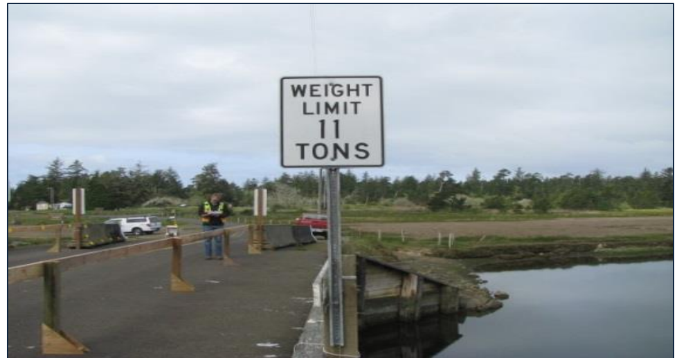
Whalen Island Bridge Posting
