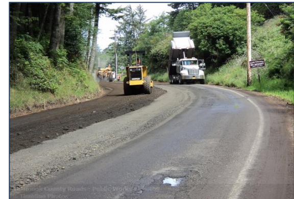
Rehabilitating Brooten Road June 2014
