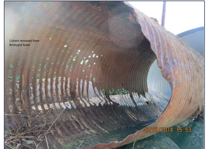
Bear Creek Culvert removed on Brickyard Road
