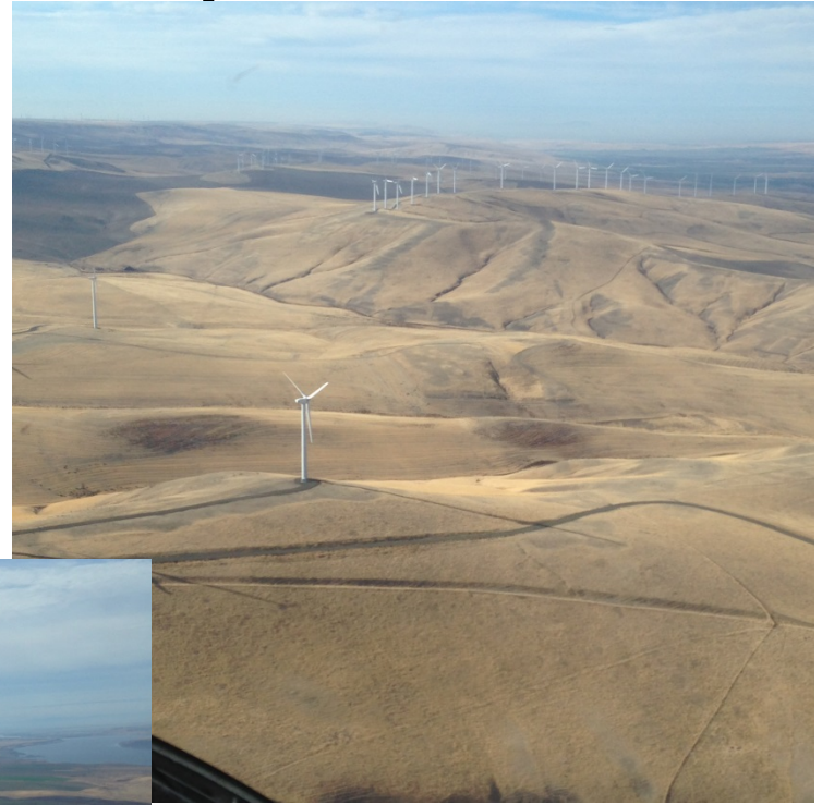
Some roads support economic development
