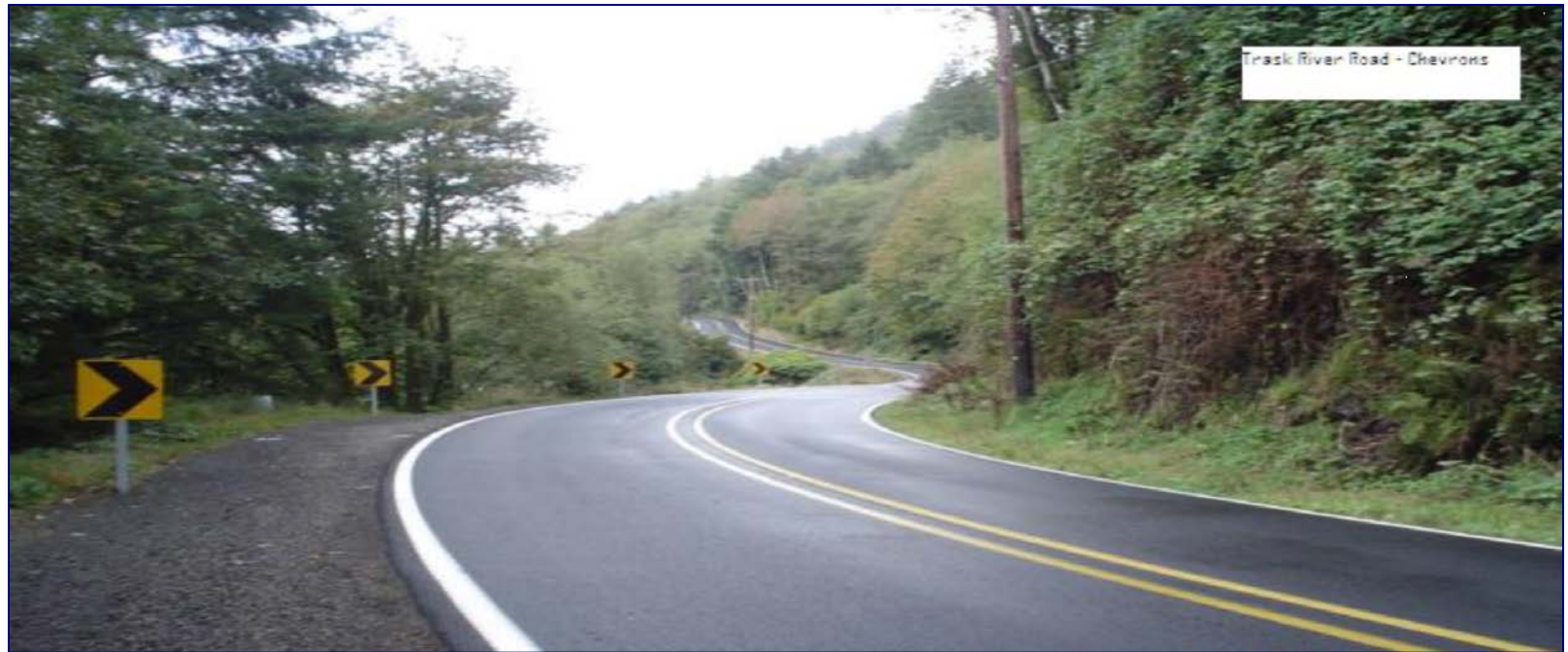
Trask River Road Signing and Striping
