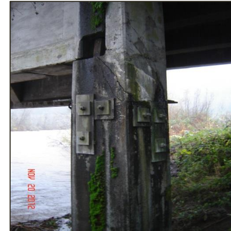
Lommen Bridge- Before
