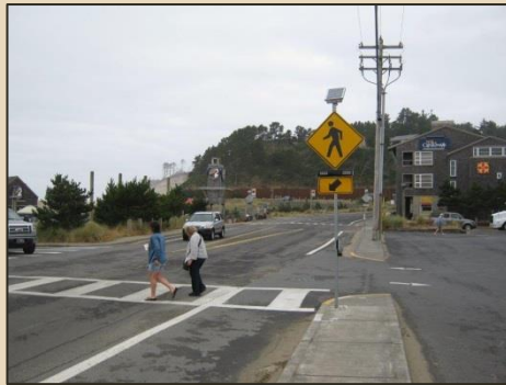
Cape Kiwanda Solar Pedestrian Lights
