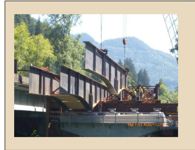
Lommen Bridge – Reconstruction almost completed
