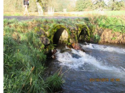
Sifford Culvert removed on Bower Creek - Before
