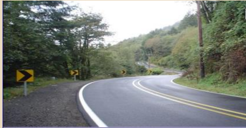
Trask River Road - Signing and Striping
