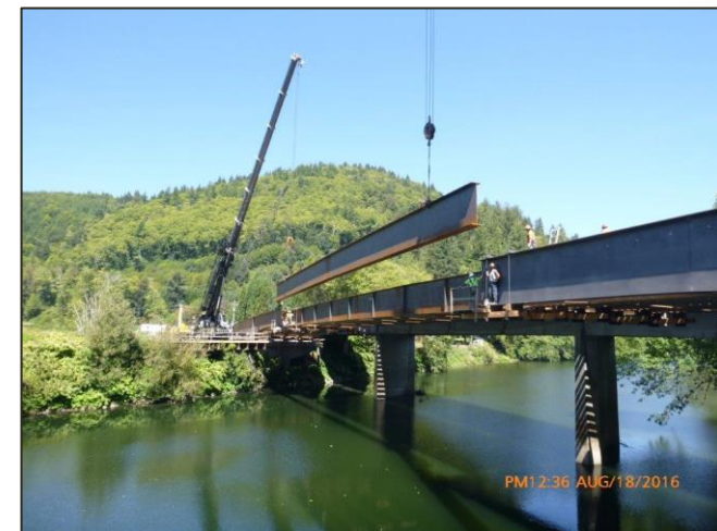
Lommen Bridge Replacement - During
