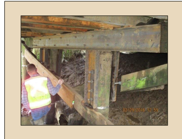
Goodspeed Bridge Rehabilitation
