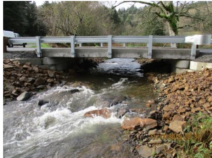
Sifford Bridge replaces a culvert
