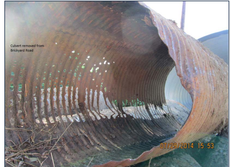
Bear Creek Culvert removed on Brickyard Road
