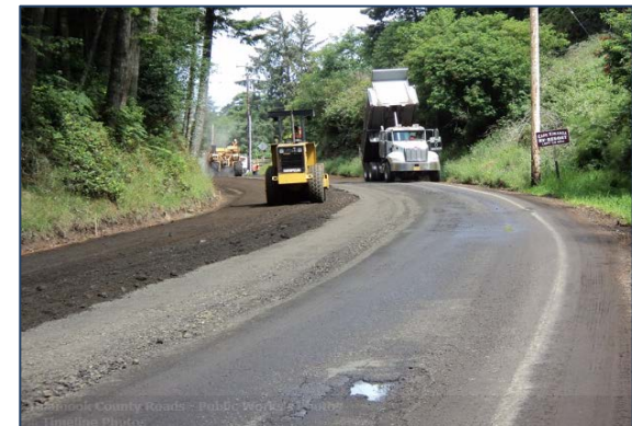
Rehabilitating Brooten Road June 2014
