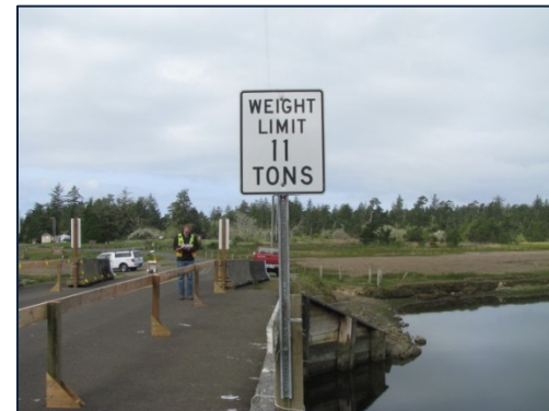
Whalen Island Bridge Posting
