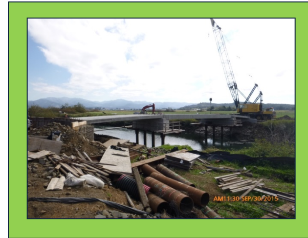
Wyss Bridge – Reconstruction almost completed
