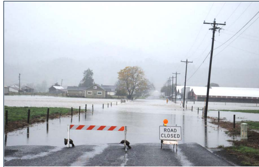
Alderbrook Road Flooding Tillamook Headlight Herald, November 2015
