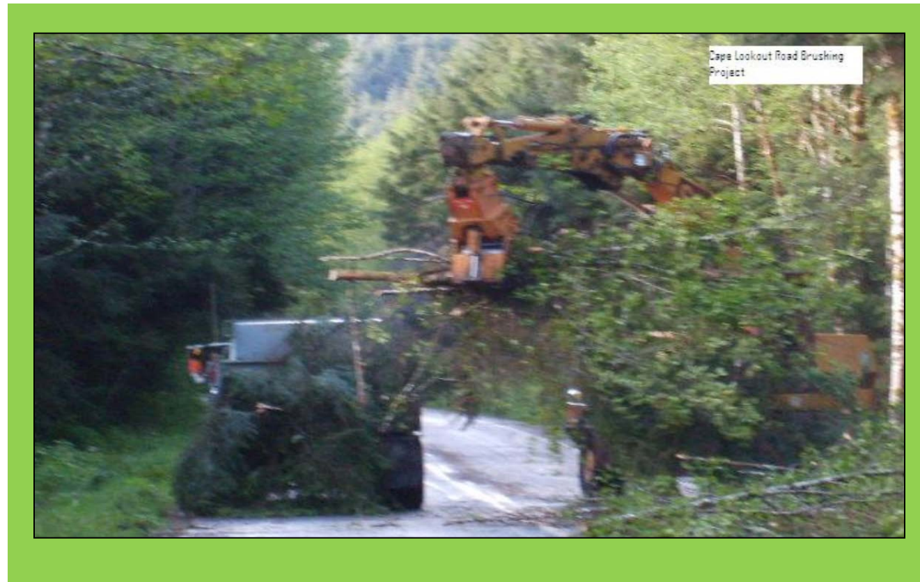
Cape Lookout Brush Cutting Project
