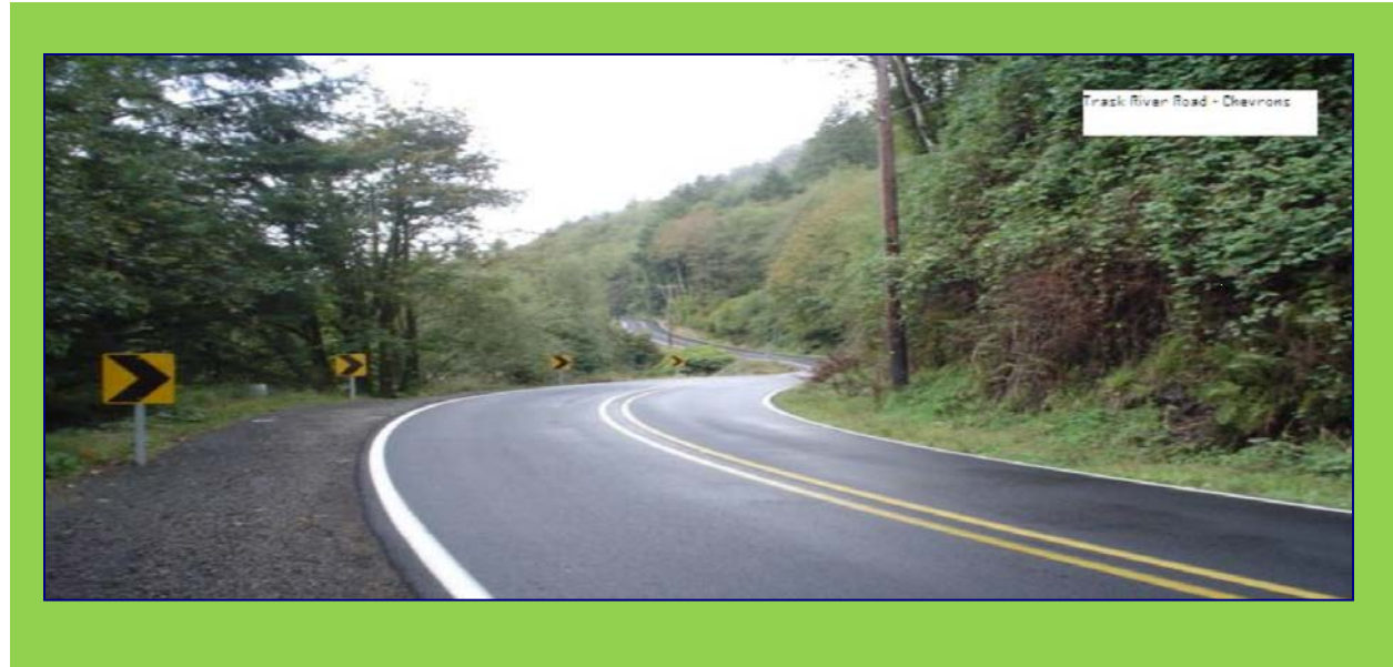
Trask River Road - Signing and Striping
