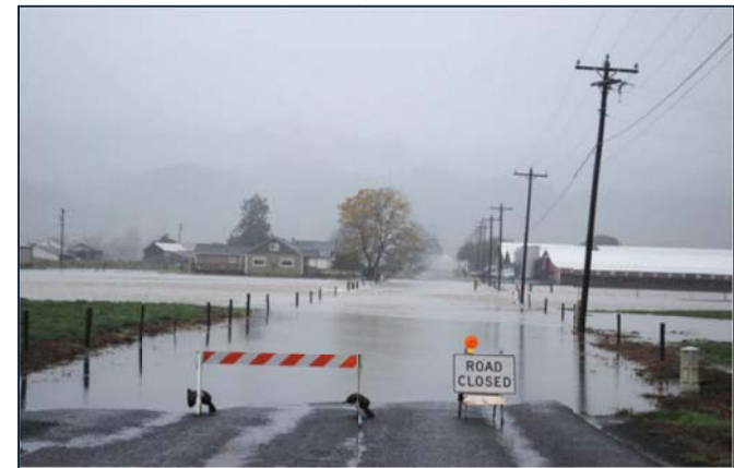
Alderbrook Road Flooding Tillamook Headlight Herald, November 2015
