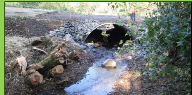
Bear Creek Culvert on Brickyard Road - After
