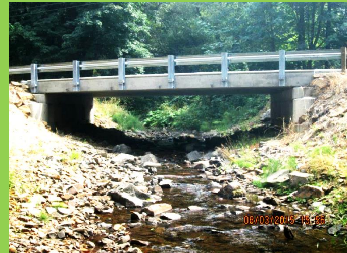
George Creek Bridge Replacement - After
