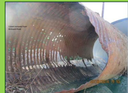
Bear Creek Culvert removed on Brickyard Road
