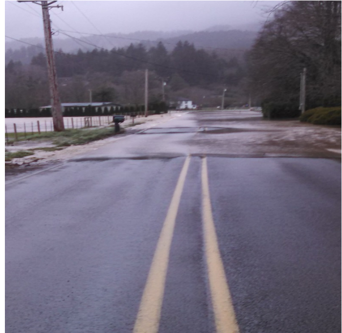
Wilson River Loop road (N-S) High Water December 2015
