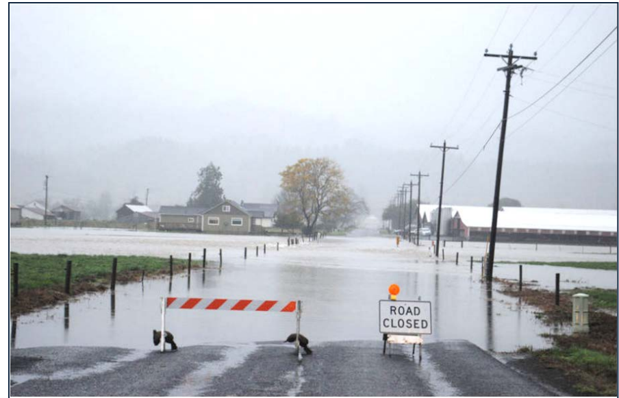
Alderbrook Road Flooding Tillamook Headlight Herald, November 2015
