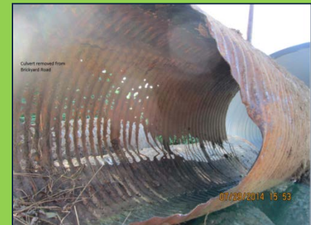
Bear Creek Culvert removed on Brickyard Road
