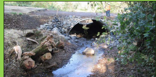
Bear Creek Culvert on Brickyard Road - After
