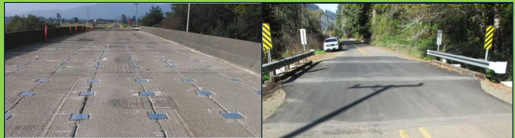
Jim Creek Bridge – Deck replaced, structure excavated, repaired & reinforced
