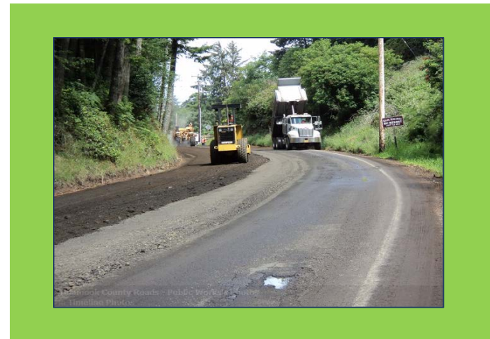
Rehabilitating Brooten Road
