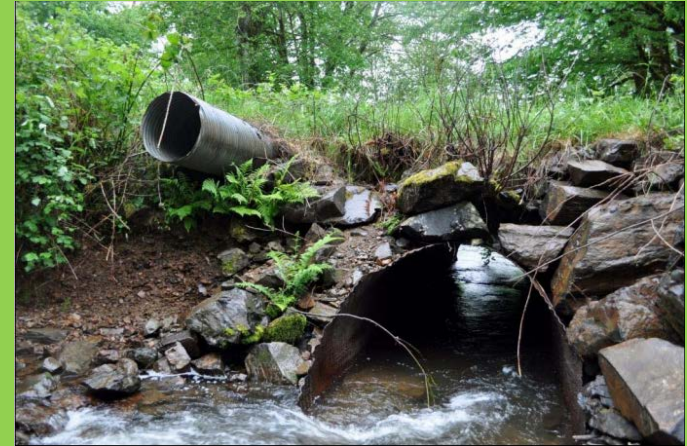
George Creek Culvert - Before
