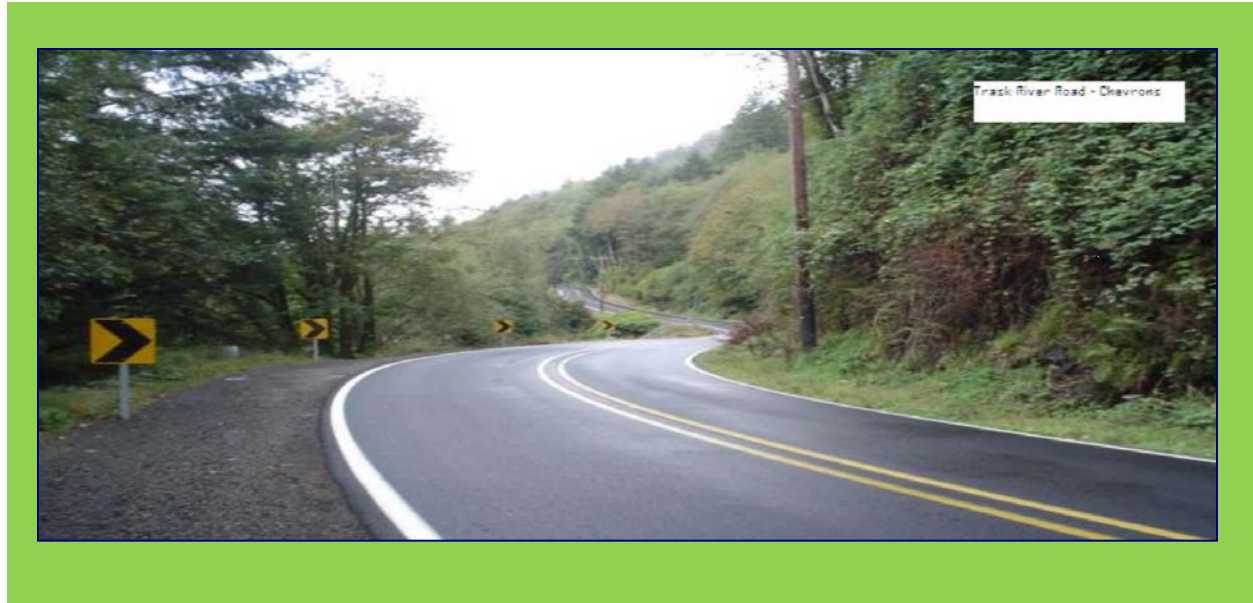
Trask River Road - Signing and Striping
