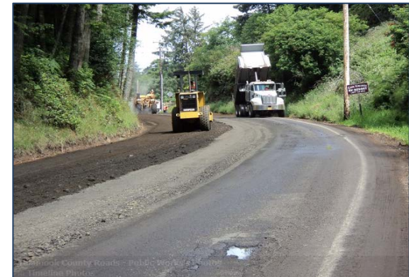
Rehabilitating Brooten Road June 2014
