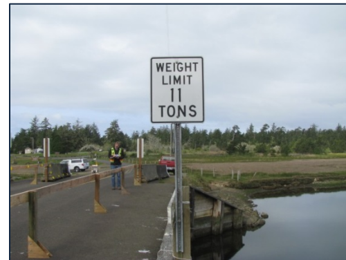
Whalen Island Bridge Posting
