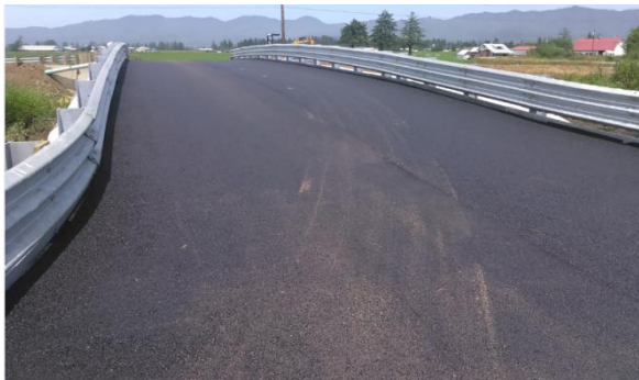
Wyss Bridge reconstruction
