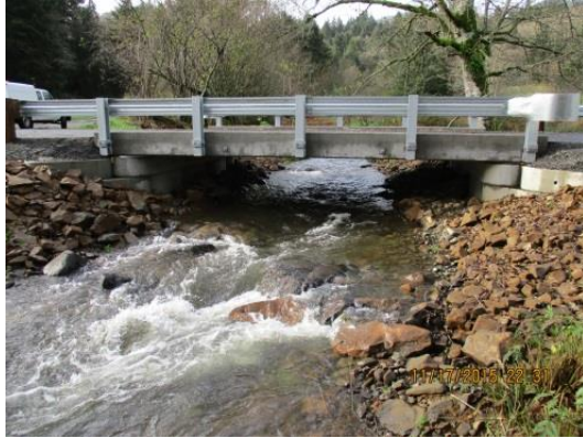
Sifford Bridge replaced a culvert in 2016
