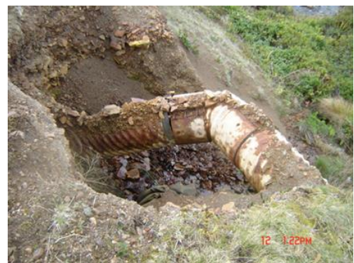
20 Sandlake Road culverts were inspected in 2017
