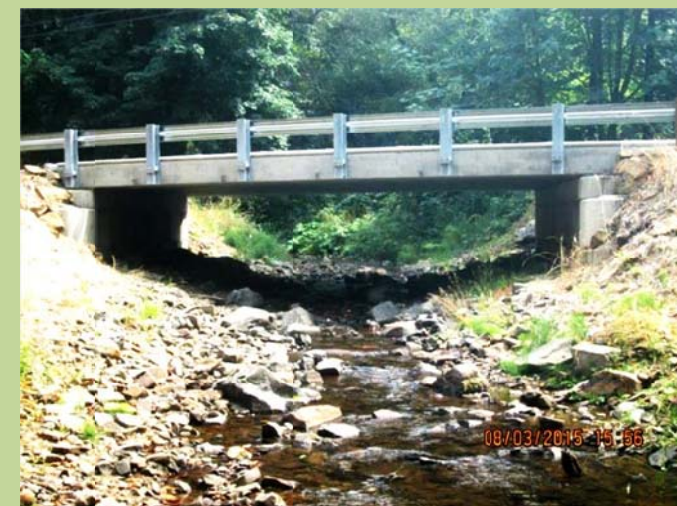
George Creek Bridge Replacement - After
