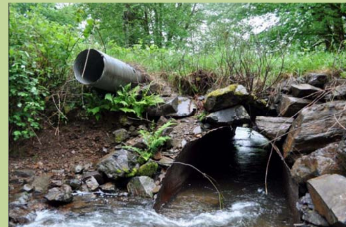
George Creek Culvert - Before
