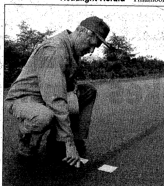
Placing temporary highway centerline markers is Mike Wynands, south district.
